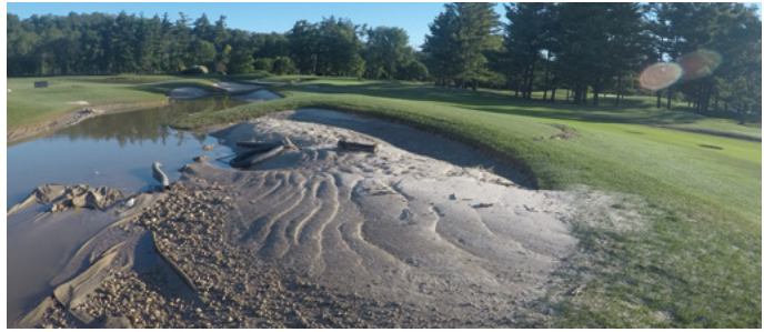
Deer Ridge #12 bunker washed out.
