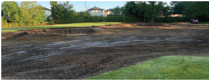
Hole #17, Rivermead, green complex during renovations work.
